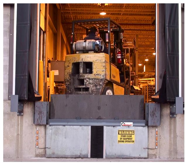
Pentalift's Series "HURS" roll-off stop lip hydraulic dock levelers feature all of the design, structural and operational benefits of Pentalift Hydraulic dock levelers, with the added safety enhancement of a roll-off stop lip.
