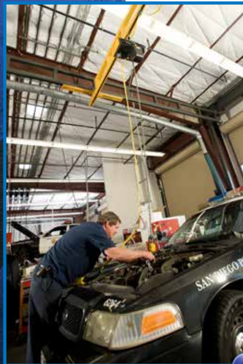
This police garage can do major maintenance tasks much easier now with a 2000-pound capacity Spanco Freestanding Bridge Crane.
